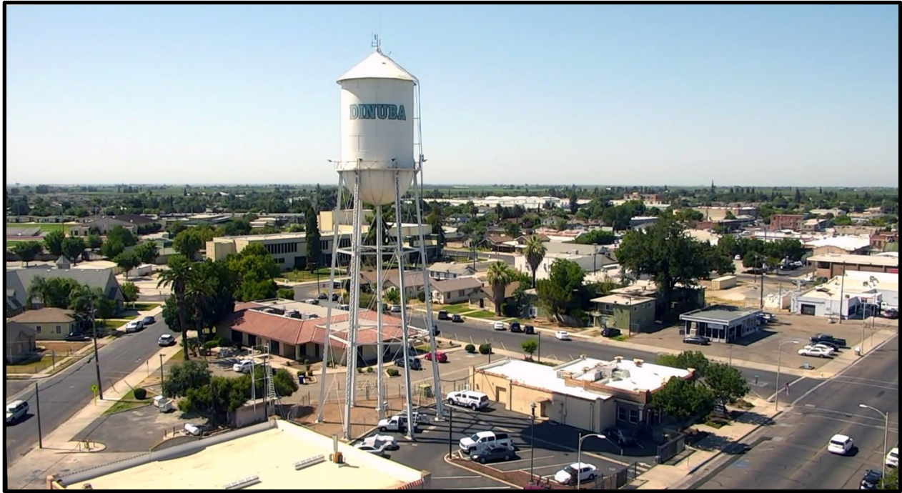
Old Dinuba Water Tower – East Tulare Street
