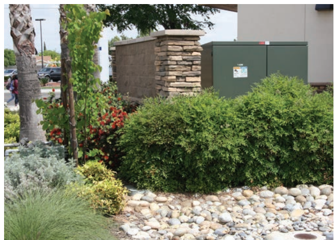
Utility Box Example
