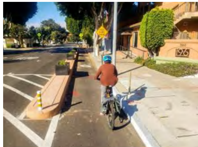
Class IV Bikeways provide a physical separation between the bikeway and adjacent traffic.
