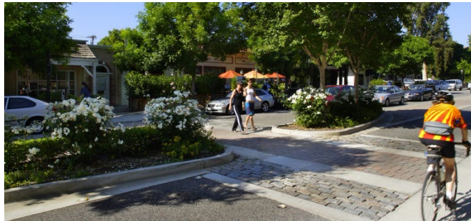
Articulated crosswalk with landscaped median & street trees
