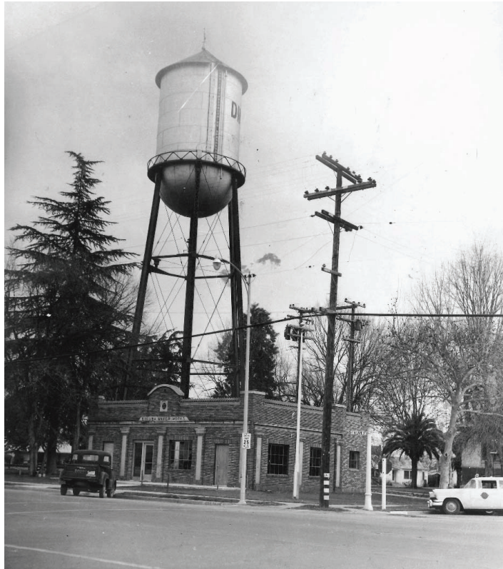
Dinuba Old Public Works Tower
